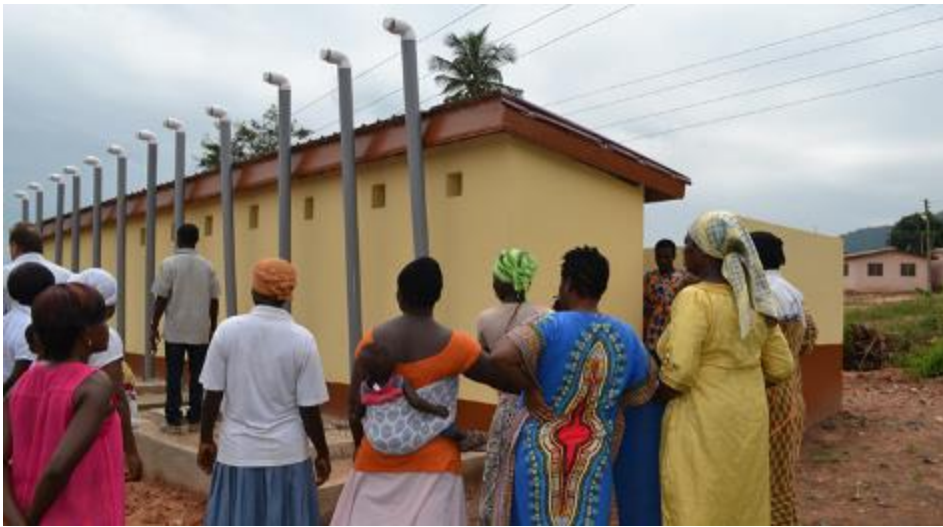
Above: community members from Kojokrom turn out to meet Council and Board Members by their newly constructed KVIP latrine
