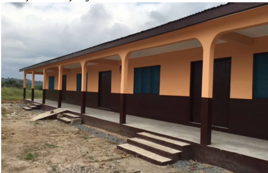
Above: the new classroom block for Pampanso Primary School.
