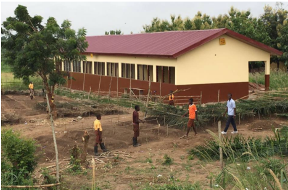
Above: The new classroom block at Kyinto Junior High School with their school farm in the foreground.
